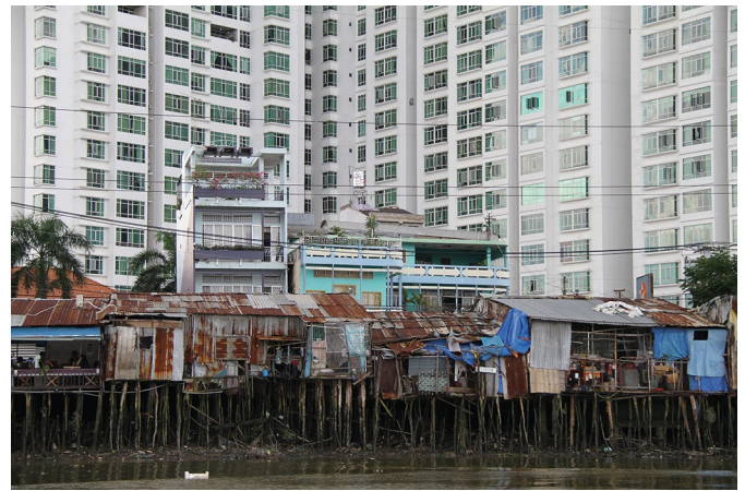
Fig. 3 | Stilt houses on a river bank in Ho Chi Minh City, Vietnam. This flood-mitigation measure is widely applied by the poorest, most exposed and most vulnerable part of the population and stands in stark contrast to the new high-rise residential apartments in the background. Credit: Stijn Koole, Bosch Slabbers Landscape + Urban Design.
