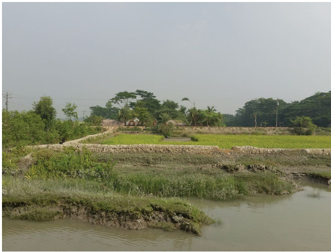
Fig. 2 | Polder system in coastal Bangladesh south of Khulia. Polders are low-lying tracts of land enclosed by dikes, which are widespread in densely populated deltas with the main goal of promoting agriculture. The polder dikes and drains will require substantial upgrades to remain effective under SLR.
