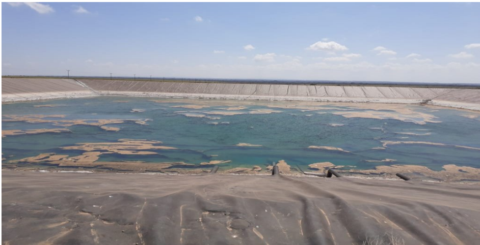
Figure 5: One of the Giant Reservoirs of PT MSM. Photograph by SP1.
